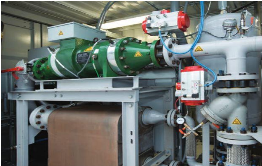
Figure 19. The Calnetix 125 MT Thermapower® ORC unit
